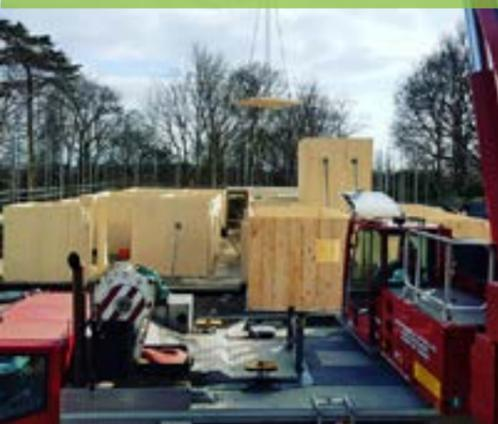
The frame production was then fabricated off-site and installed on-site. Therefore, the need for cutting or changes were kept to a minimum once on-site.
